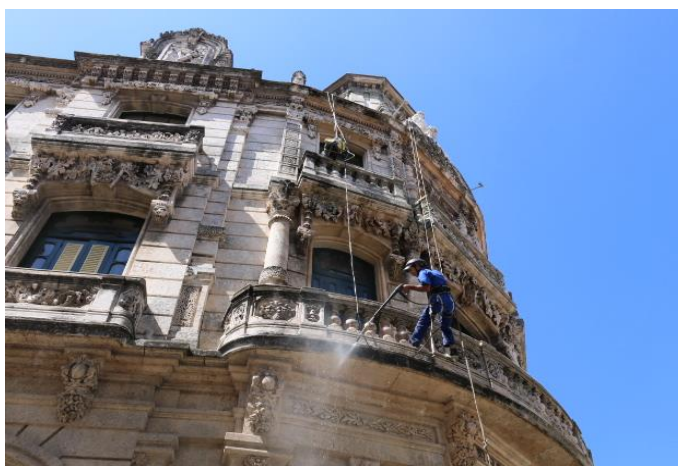
Worker washes down Old Havana building.
